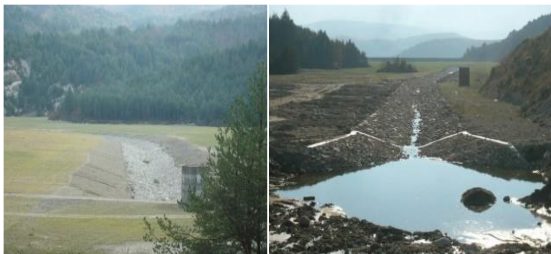
Fig. 2. Engineering activity on the closure of Eleshnitsa Mine
